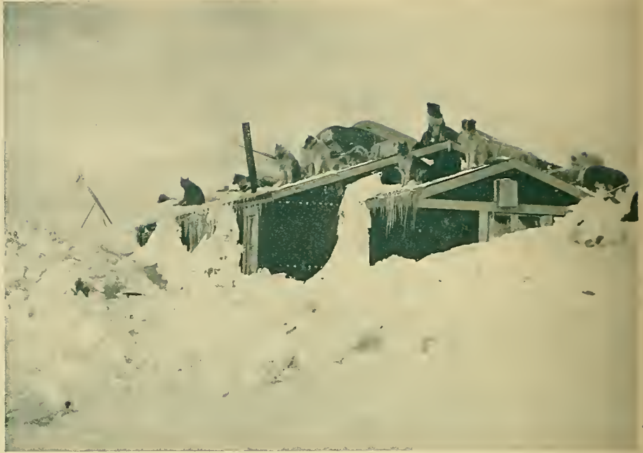
THE APPEARANCE OF THE HUT ON THE RETURN OF LIGHT IN 1905
